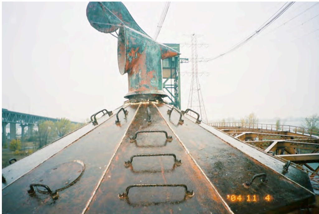
Detail of top of lantern showing ventilator with wind vane, which keeps the vent pointing downwind.
