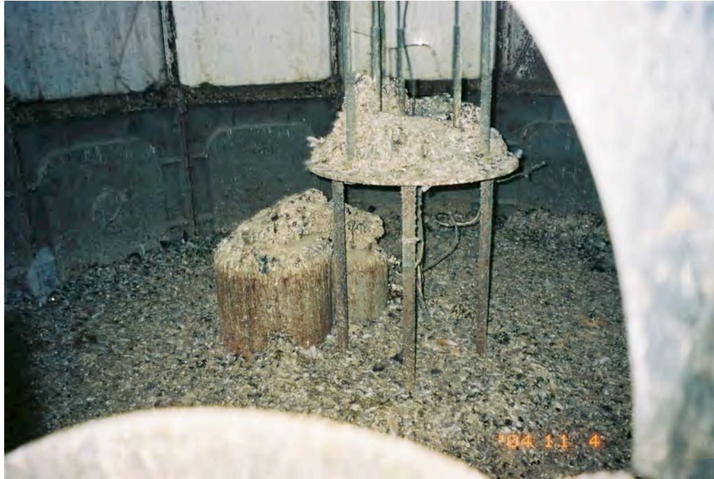
Detail of floor of lantern. Note the depth of guano on the floor. This material contains fungus and can be toxic to humans.
