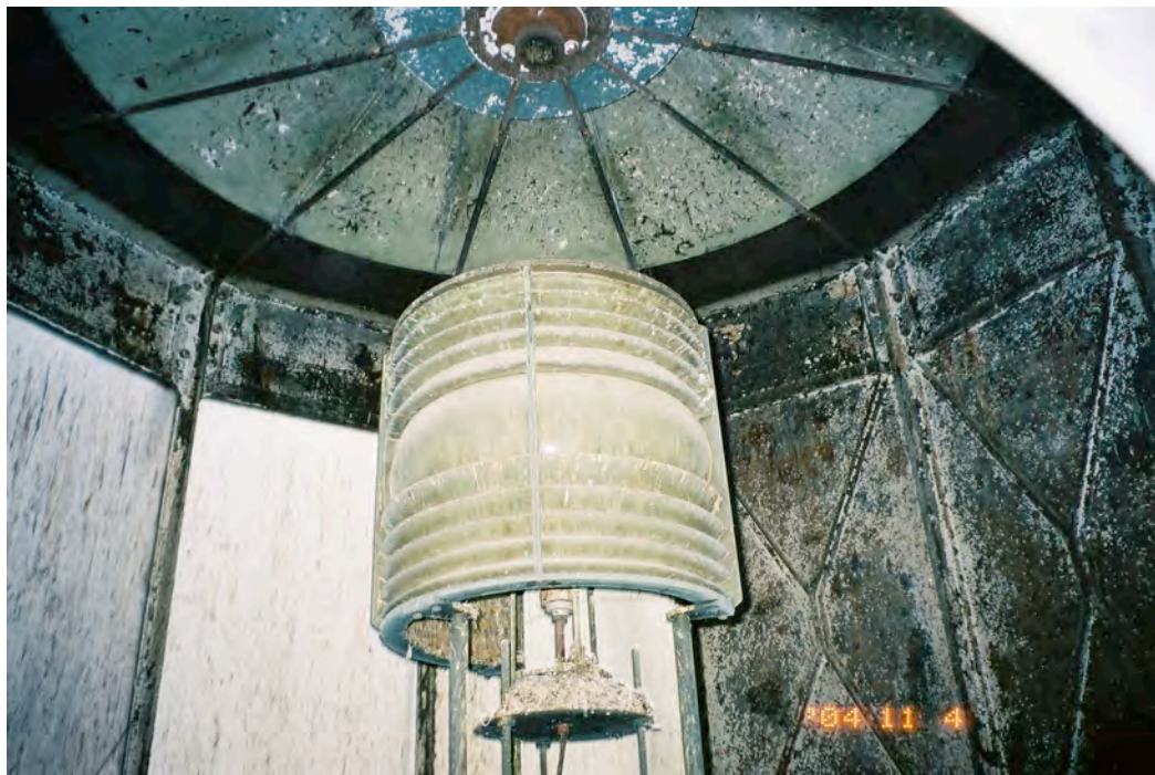
Image of last beacon mounted inside the lantern. This beacon is electric and is a mid-20 th century replacement for the earlier lights
