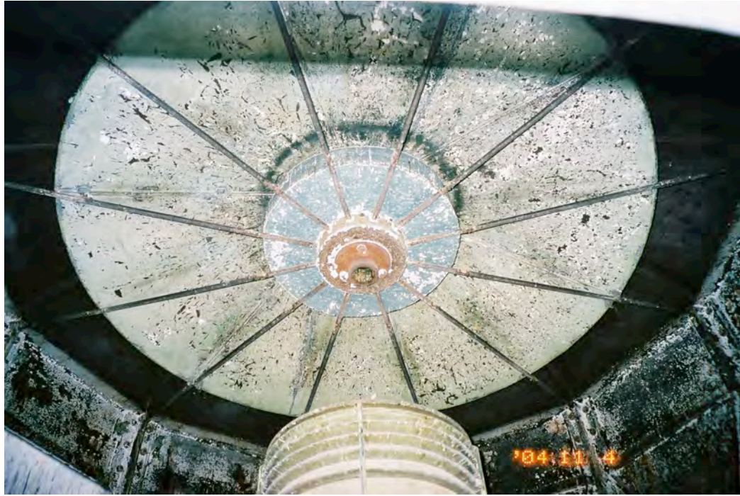
Detail of the underside of the roof of the lantern. The details suggest an early 20 th century design, which would have replaced an earlier 1850's assembly. Further research should be done.
