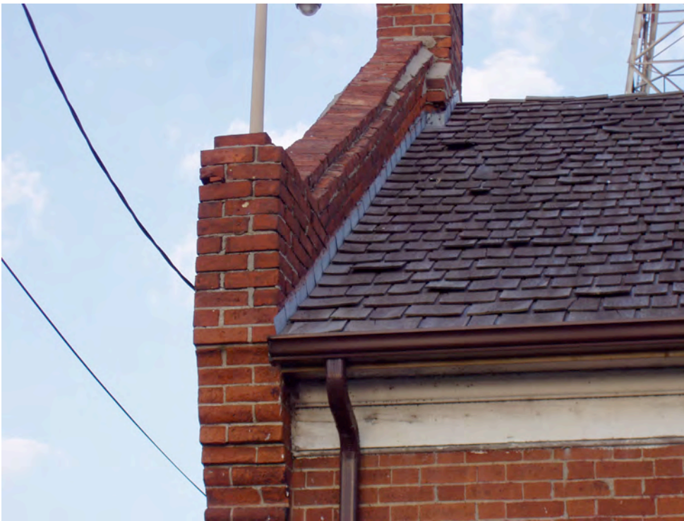
Detail of north gable. Note the shoulder under the chimney, which is the base of the original chimney.
